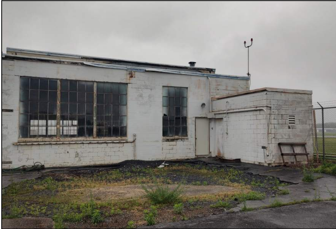
1. View of the D Side (East) of the Fire Station.
