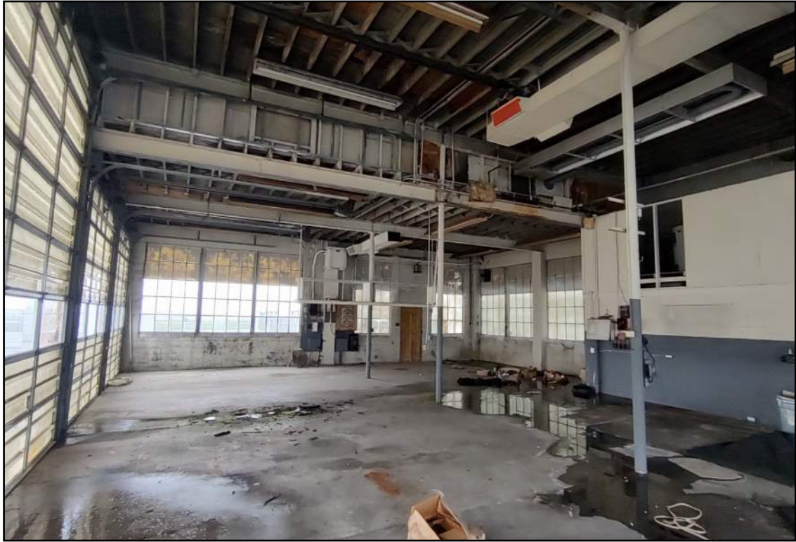
3. View of the interior of the Fire Station.
