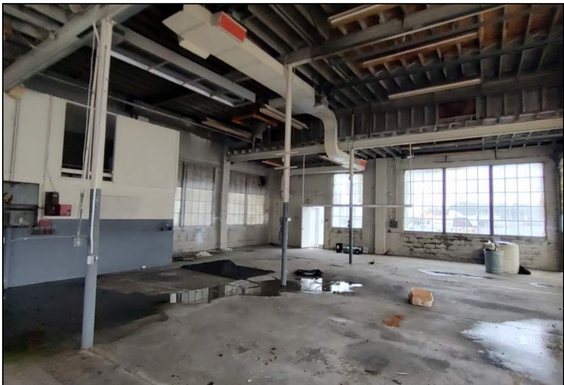
4. View of the interior of the Fire Station.
