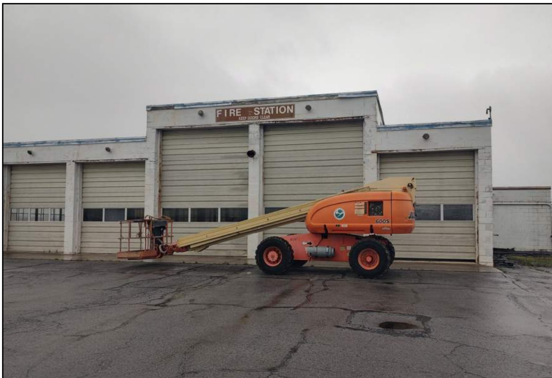
2. View of the A Side (South) of the Fire Station.
