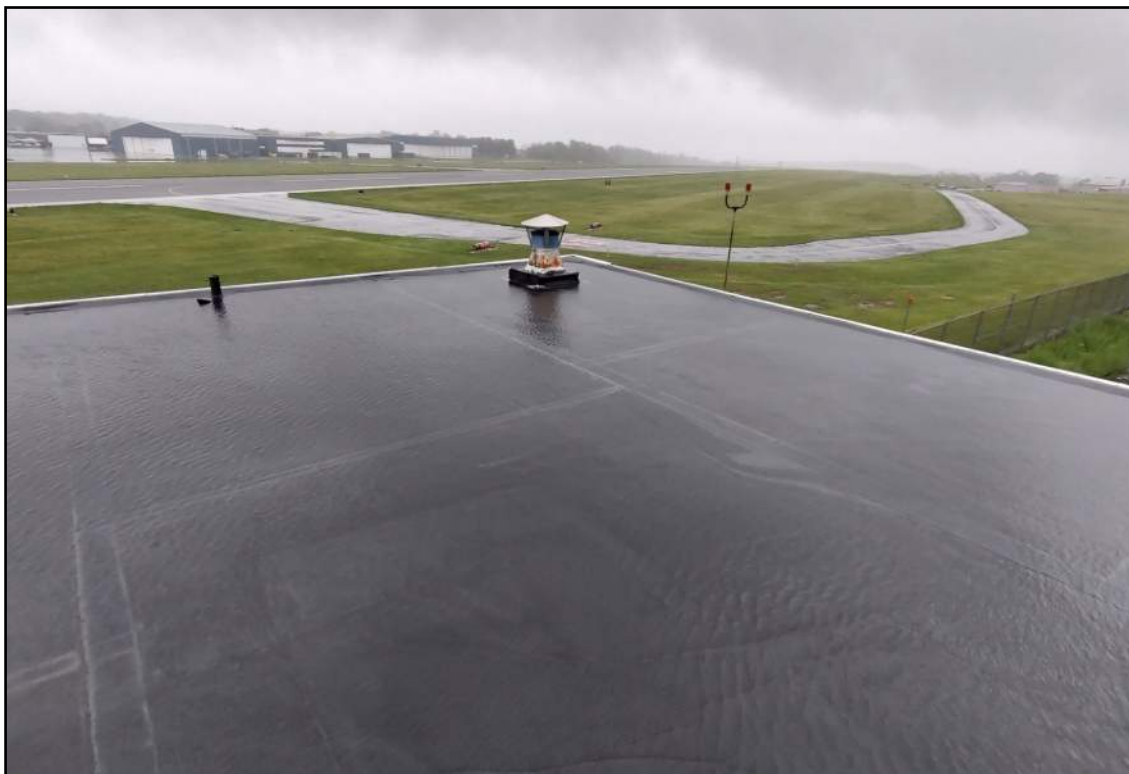
10. View of vent and exhaust pipes on the Roof.
