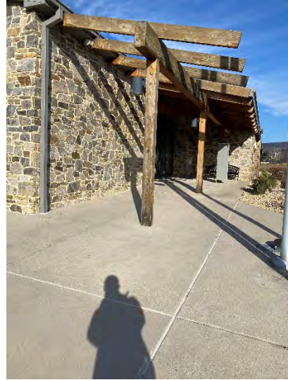
Exterior Entrance Route
