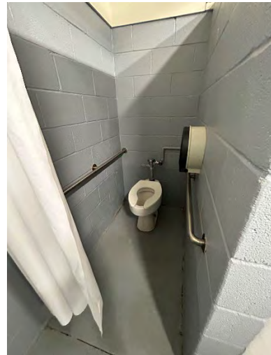
Pool Men's Toilet Room Accessible Water Closet / Stall
