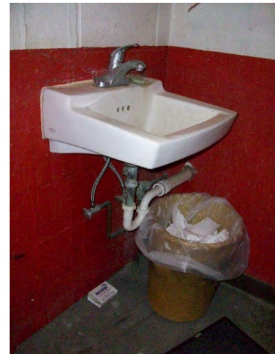
Toilet Room Sink
