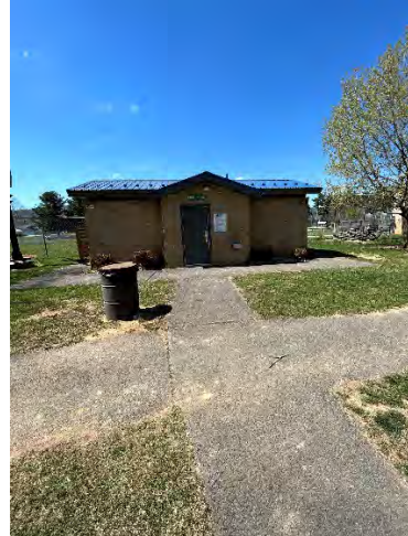
Pathway to Toilet Rooms
