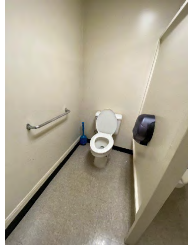
Men's Toilet Room Accessible Water Closet / Stall
