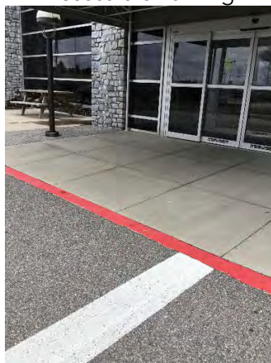
Exterior Entrance Route
