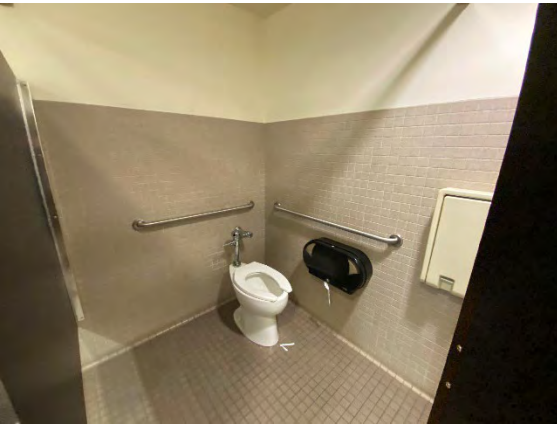
Men's Toilet Room Accessible Water Closet / Stall
