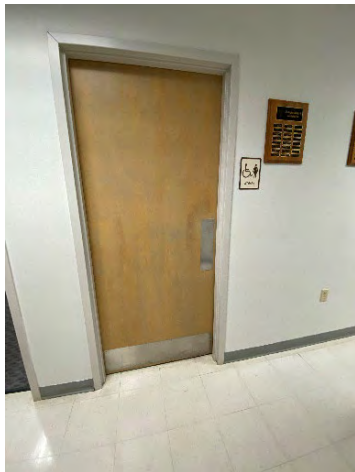
Women's Toilet Room Entrance
