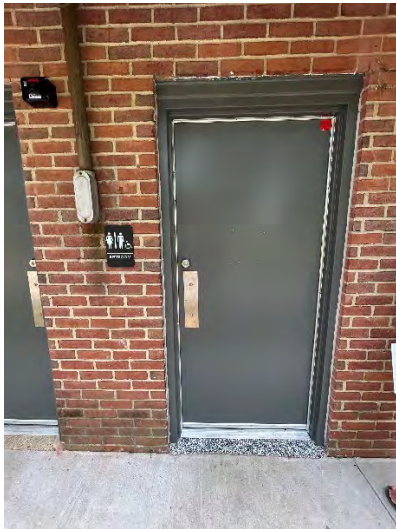
Northern Pavilion Right/West Toilet Room Entrance
