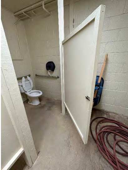
Men's Toilet Room Accessible Stall
