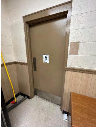
Rear Men's Toilet Room Entrance
