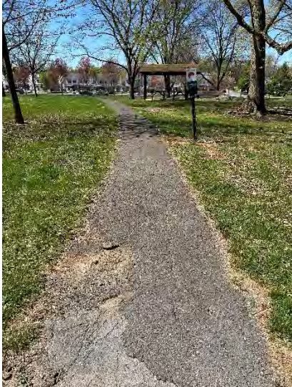
Exterior Entrance Route from Woodland Way
