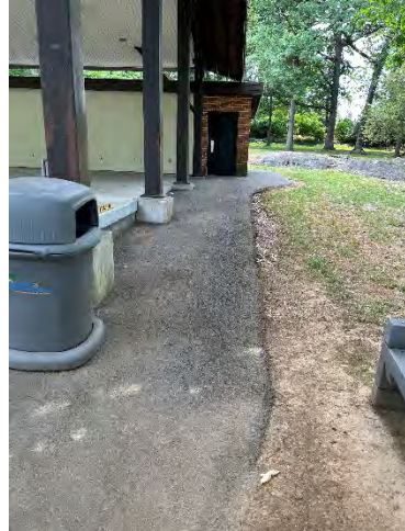
Arts Pavilion Ramp (North Side)
