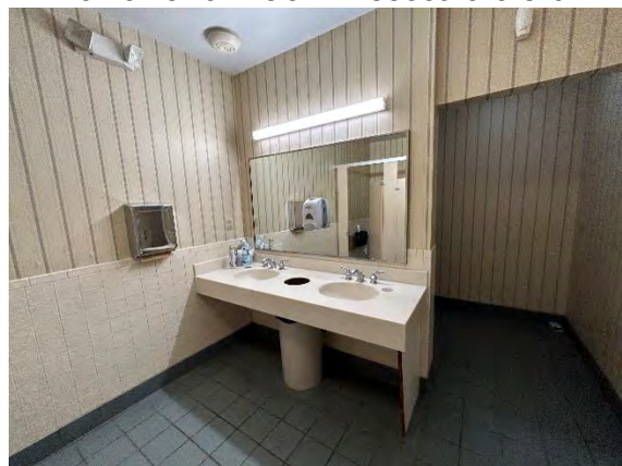
Women's Toilet Room Sink / Route
