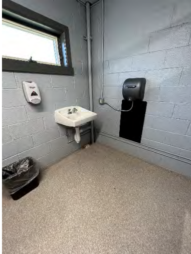
Pavilion #1 Women's Toilet Room Sink
