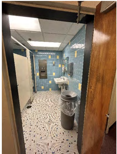
3 rd Floor Women's Toilet Room Interior
