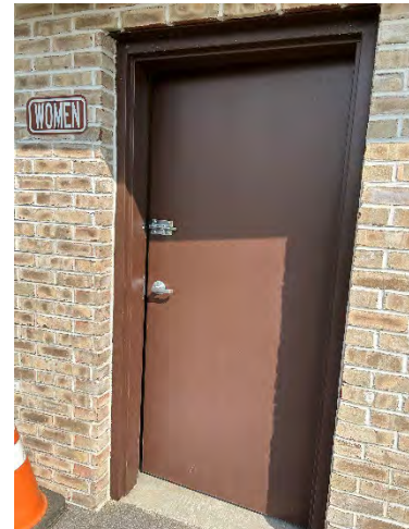
Women's Toilet Room Entrance
