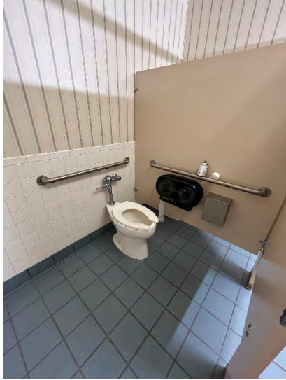
Women's Toilet Room Accessible Stall
