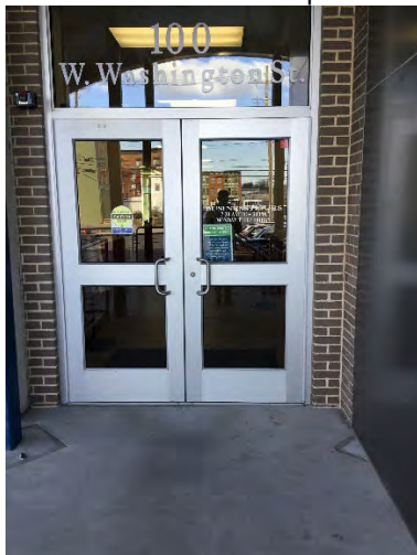
Entrance (From Parking Lot)
