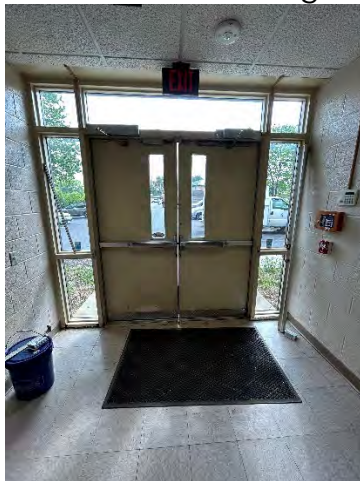
Main Entrance Interior
