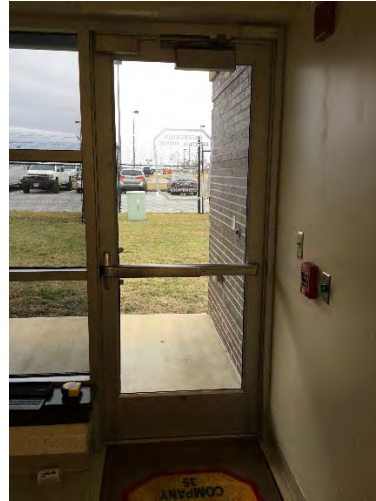
Main Entrance Interior
