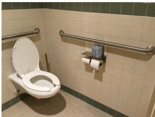
Women's Toilet Room Accessible Water Closet / Stall
