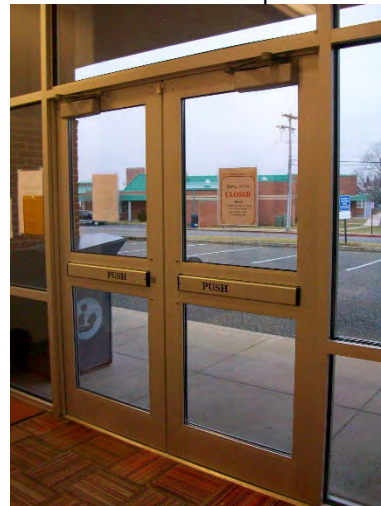
Main Entrance Interior
