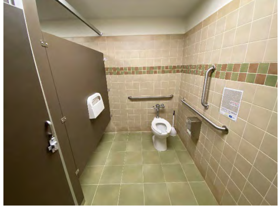
Women's Toilet Room Accessible Water Closet / Stall
