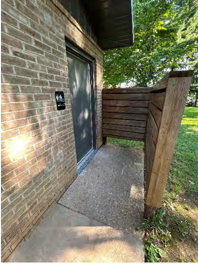
Tennis Court Right Toilet Room Entrance
