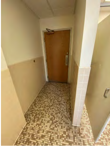
3 rd Floor Men's Toilet Room Interior Entrance
