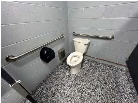
Arts Pavilion Women's Toilet Room Accessible Water Closet / Stall
