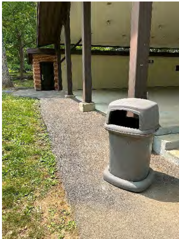
Arts Pavilion Ramp (South Side)
