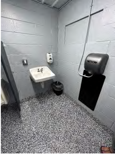
Southern Pavilion Left/North Toilet Room Sink
