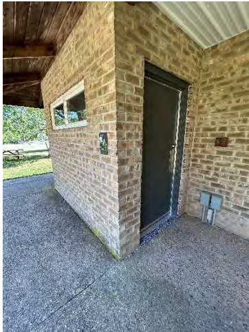
Lower Pavilion - Women's Toilet Room Entrance
