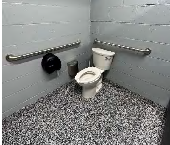
Northern Pavilion Left/East Toilet Room Accessible Water Closet / Stall
