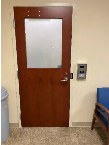
County Commissioner Office Interior / Secure Entrance
