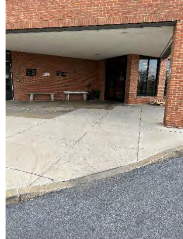
Main Entrance Route / Curb Ramp
