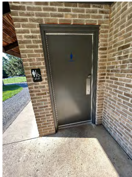
Pavilion #2 Women's Toilet Room Entrance
