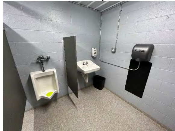
Men's Toilet Room Interior
