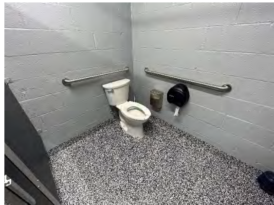
Northern Pavilion Right/West Toilet Room Accessible Water Closet / Stall
