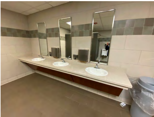
1 st Floor Men's Toilet Room Sinks
