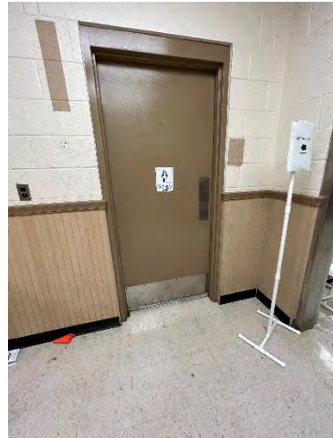
Rear Women's Toilet Room Entrance
