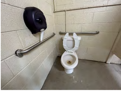
Women's Toilet Room Accessible Water Closet
