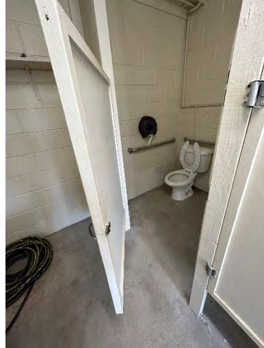
Women's Toilet Room Accessible Stall
