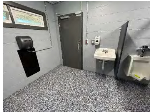
Pavilion #2 Men's Toilet Room Sink
