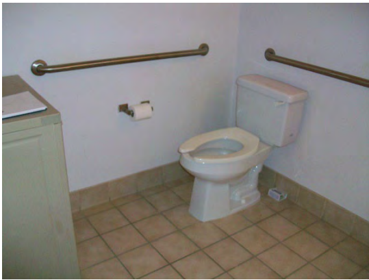
Women's Toilet Room Water Closet
