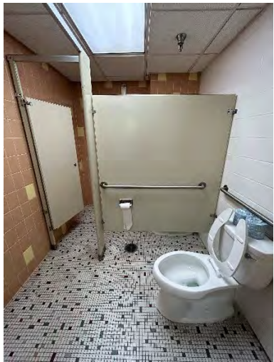
3 rd Floor Men's Toilet Room Accessible Water Closet / Stall
