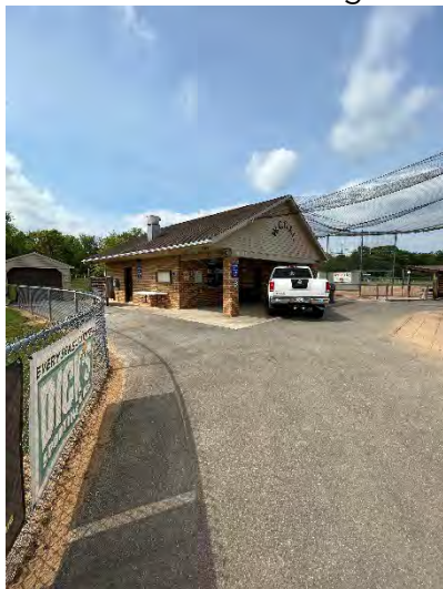
Pathway / Main Building
