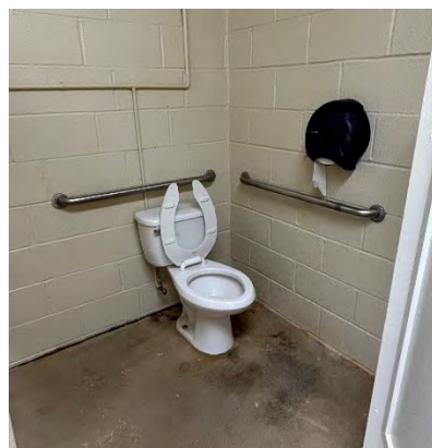
Men's Toilet Room Accessible Water Closet
