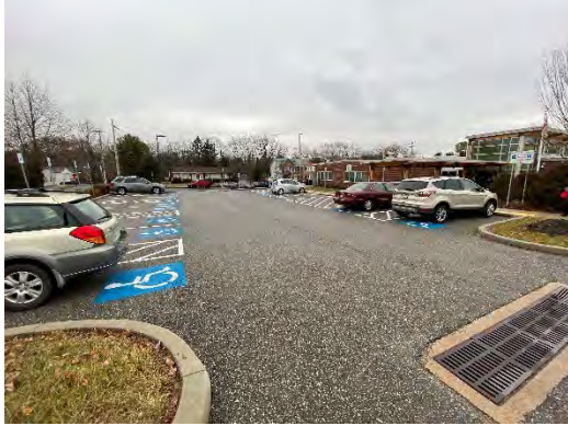
Front Parking Lot Accessible Parking
