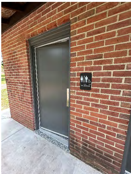
Northern Pavilion Left/East Toilet Room Entrance
