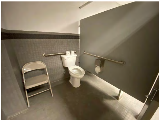
Men's Toilet Room Accessible Water Closet / Stall
