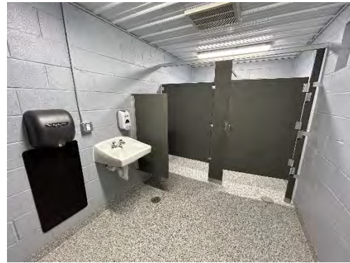
Men's Toilet Room Interior
