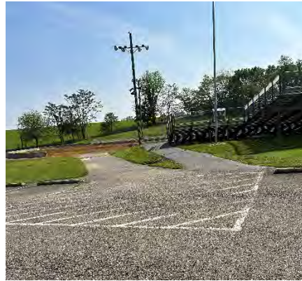
Access Aisle & Exterior Accessible Route
