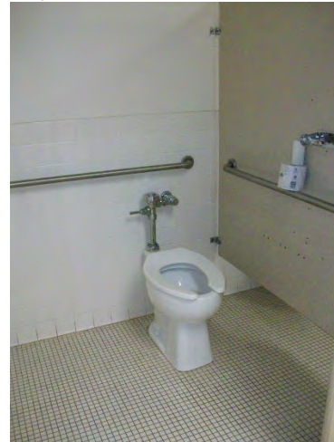
(Left) Men's Toilet Room Accessible Water Closet / Stall
