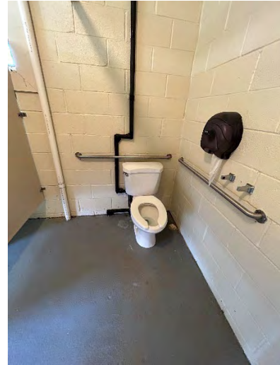
Women's Toilet Room Accessible Water Closet / Stall
