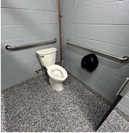
Arts Pavilion Men's Toilet Room Accessible Water Closet / Stall
