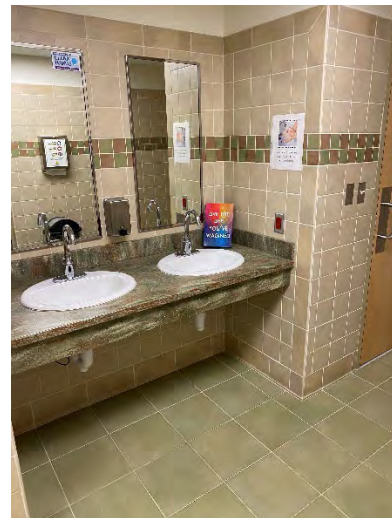
Men's Toilet Room Sinks
