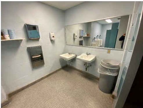
2 nd Floor Men's Toilet Room Sinks
