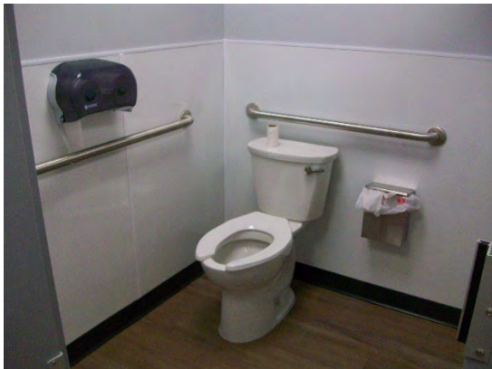
Women's Toilet Room Accessible Water Closet / Stall
