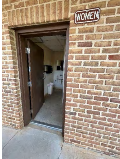
Women's Toilet Room Entrance
