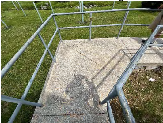
Ramp Turning Area
