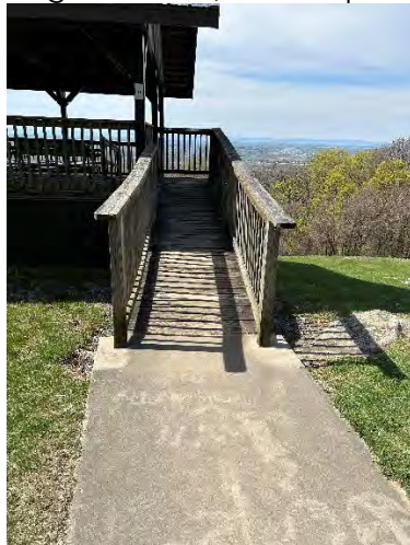
Ramp Entrance to Overlook Structure
