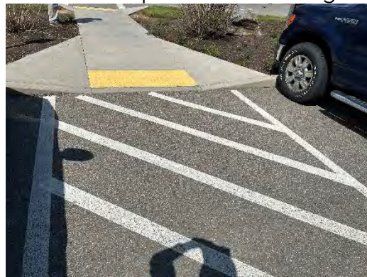
Curb Ramp at Access Aisle
