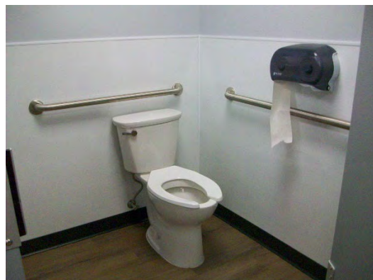
Men's Toilet Room Accessible Water Closet / Stall
