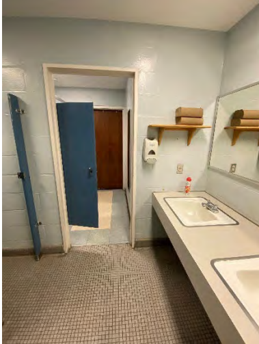
3 rd Floor Women's Toilet Room Interior
