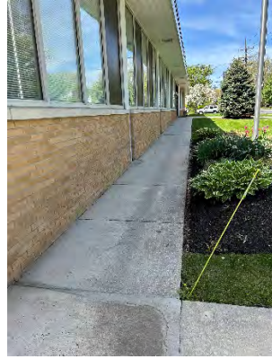
Exterior Entrance Route
