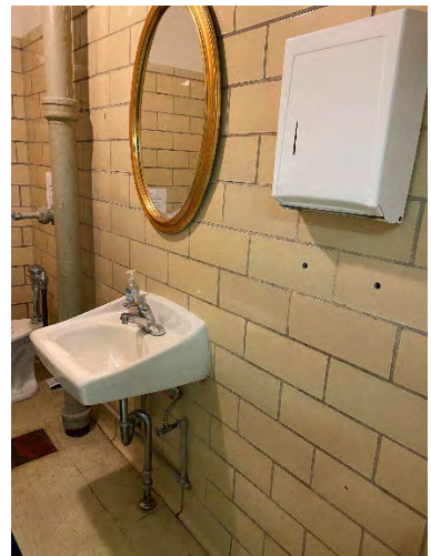
Single-Use Toilet Room Sink
