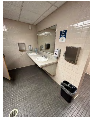
1 st Floor Men's Toilet Room Sinks
