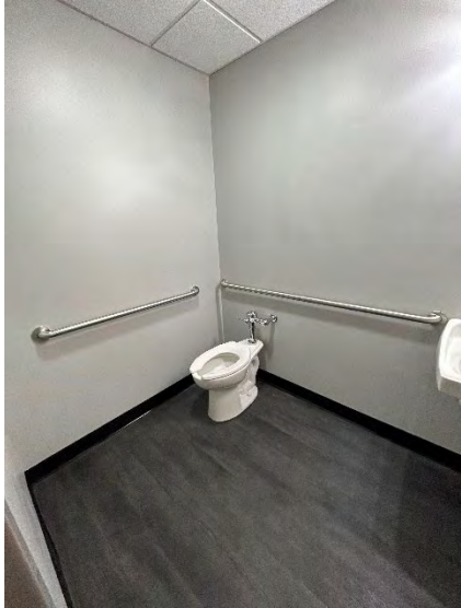
Accessible Toilet Room Water Closet
