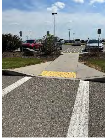
Curb Ramp at Road Crossing
