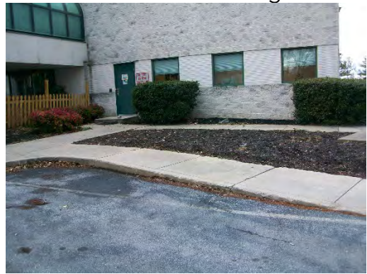
Exterior Entrance Route
