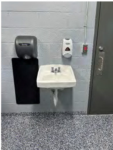
Lower Pavilion - Women's Toilet Room Sink
