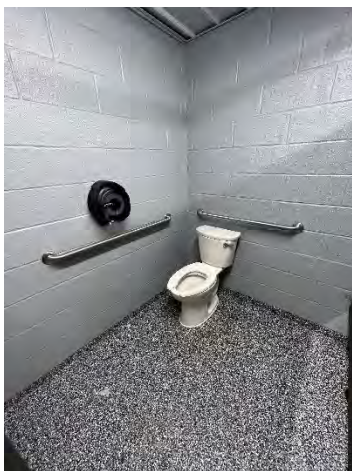
Men's Toilet Room Accessible Water Closet / Stall
