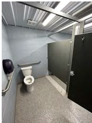
Men's Toilet Room Accessible Water Closet / Stall
