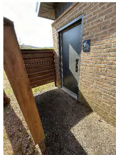
Women's Toilet Room Entrance
