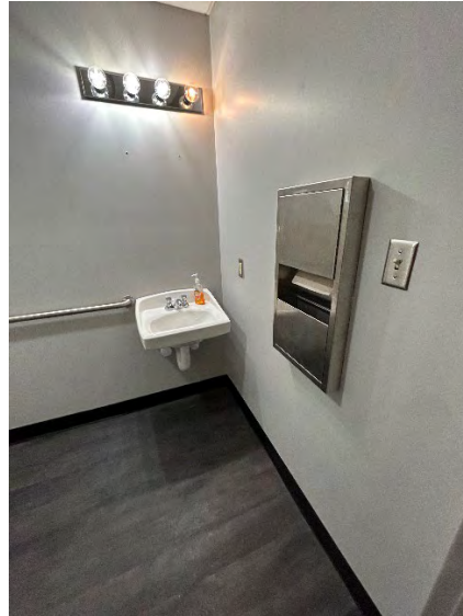
Accessible Toilet Room Sink
