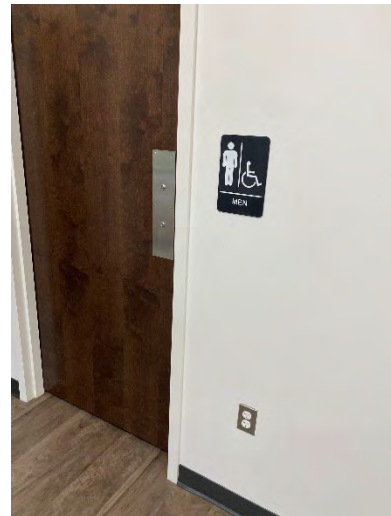
Men's Toilet Room
