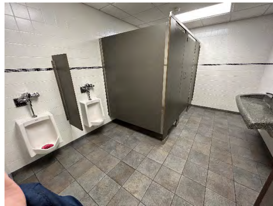
2 nd Floor Men's Toilet Room Interior
