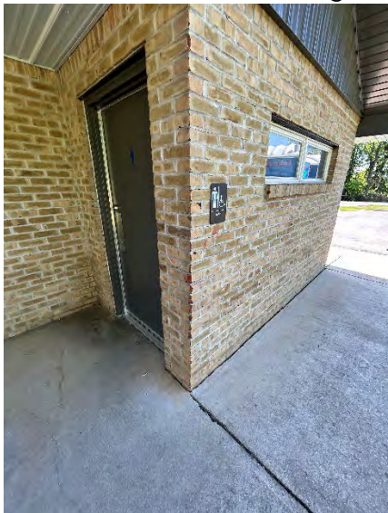
Pavilion #3 Men's Toilet Room Entrance
