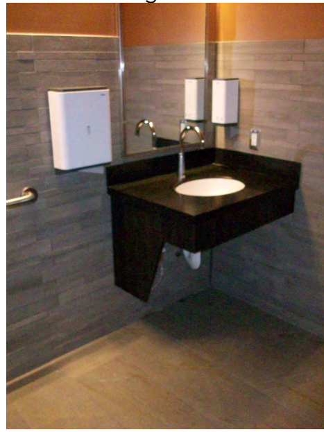
Single-Use Toilet Room Sink
