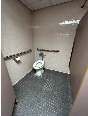
2 nd Floor Men's Toilet Room Accessible Water Closet / Stall
