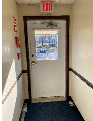
Alternative Entrance Interior
