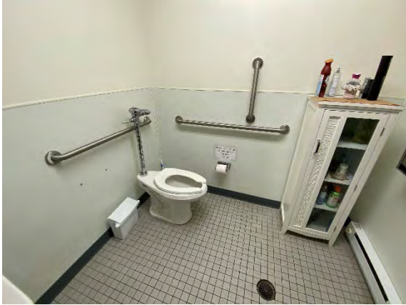
Women's Toilet Room Water Closet
