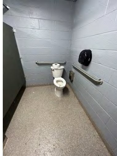
Women's Toilet Room Accessible Water Closet / Stall
