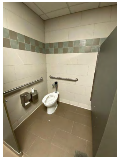
1 st Floor Women's Toilet Room Accessible Stall
