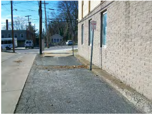
Exterior Entrance Route
