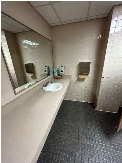
2 nd Floor Men's Toilet Room Sink
