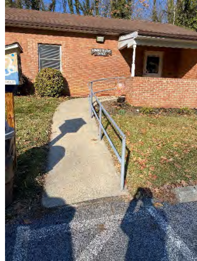
(Right) Ramp to Main Entrance
