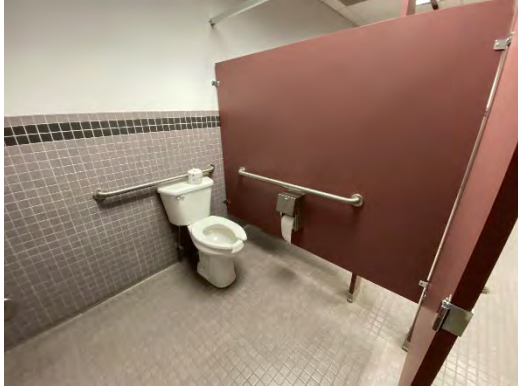
Women's Toilet Room Accessible Water Closet / Stall
