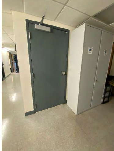
Women's Toilet Room Entrance
