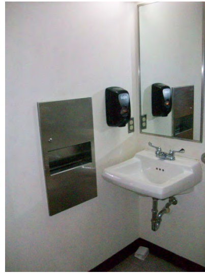
Toilet Room Sink
