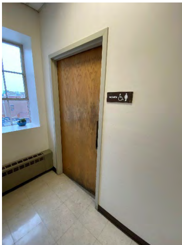
3rd Floor Women's Toilet Room Entrance
