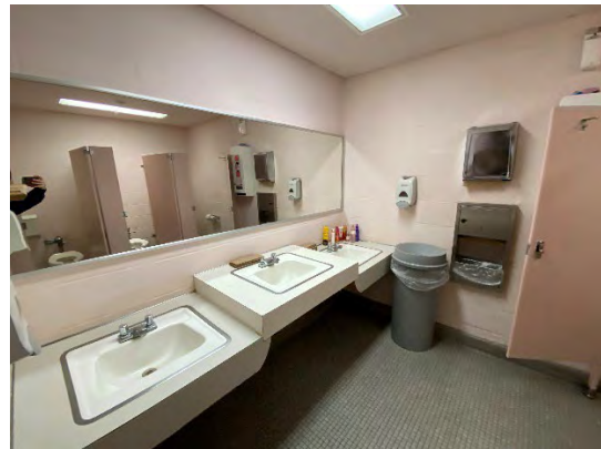
2 nd Floor Women's Toilet Room Sinks
