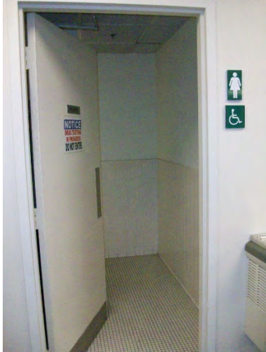
(Right) Women's Toilet Room Entrance
