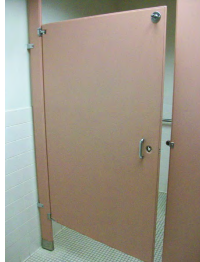
(Right) Women's Toilet Room Accessible Stall Door
