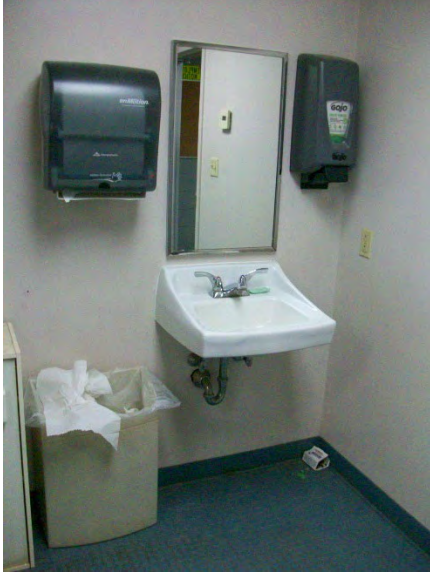
Toilet Room Sink
