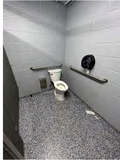
Women's Toilet Room Accessible Water Closet / Stall
