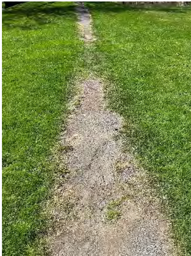
Exterior Accessible Route (To Bridge) - Close Up
