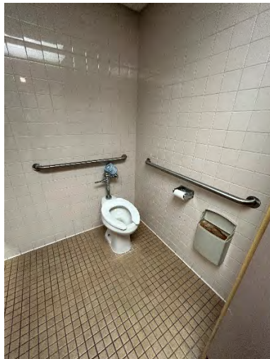
1 st Floor Women's Toilet Room Accessible Water Closet / Stall
