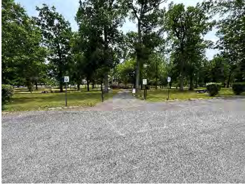
North Accessible Parking Location
