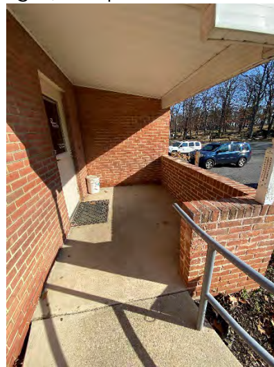
Main Entrance Exterior
