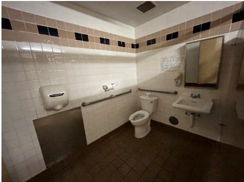
Rear Men's Toilet Room Accessible Stall
