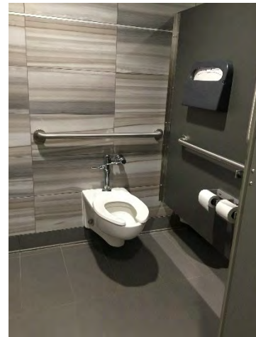
Women's Toilet Room Accessible Water Closet / Stall
