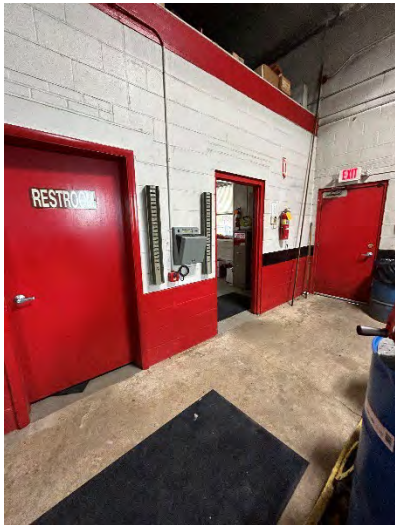
Interior Access Route
