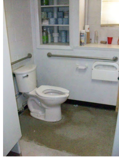
Toilet Room Accessible Water Closet / Stall
