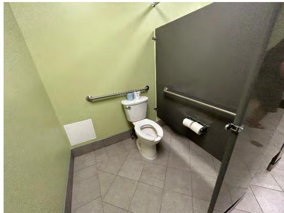
Front Men's Toilet Accessible Stall
