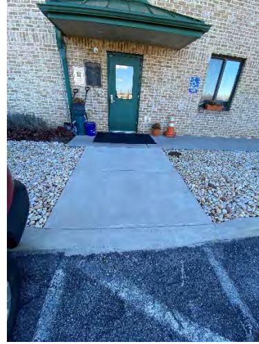
Exterior Entrance Route
