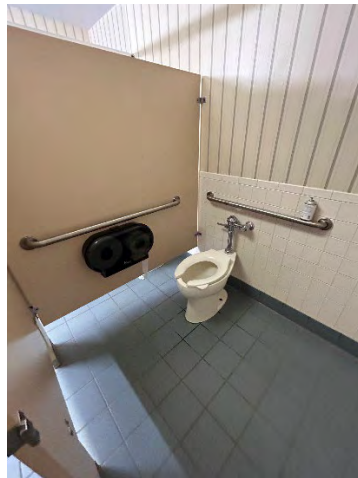
Men's Toilet Room Accessible Stall
