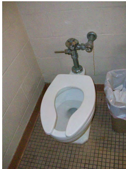
Women's Toilet Room Water Closet
