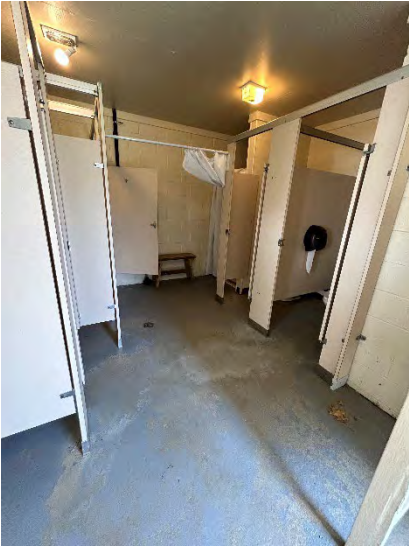
Women's Toilet Room Interior
