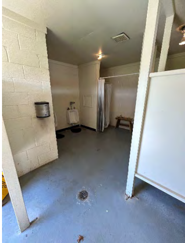
Men's Toilet Room Interior
