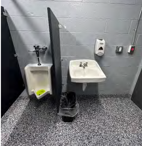
Northern Pavilion Left/East Toilet Room Sink
