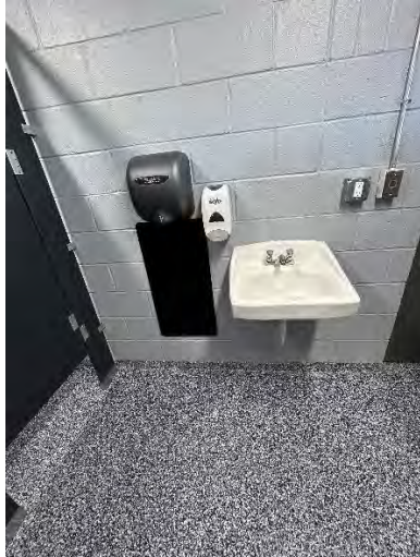
Pavilion #4 Women's Toilet Room Sink
