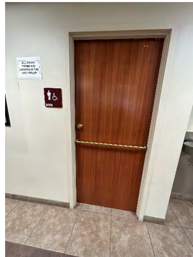
1 st Floor Men's Toilet Room Entrance
