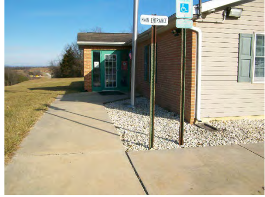
Exterior Entrance Route
