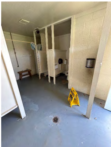
Women's Toilet Room Interior
