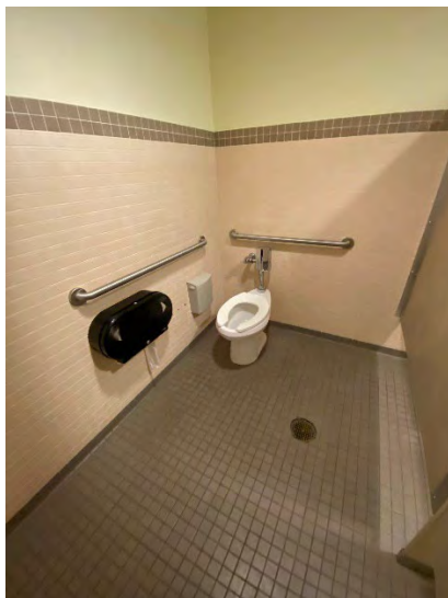
Women's Toilet Room Accessible Water Closet / Stall
