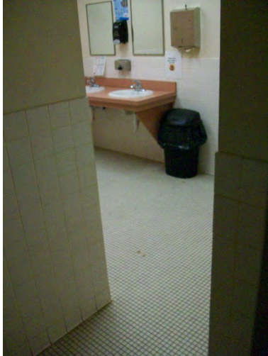
(Left) Women's Toilet Room Interior Access Route
