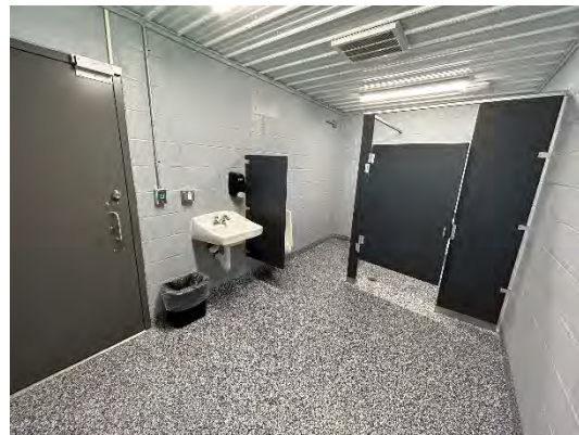
Men's Toilet Room Interior
