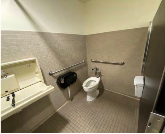
Women's Toilet Room Accessible Water Closet / Stall
