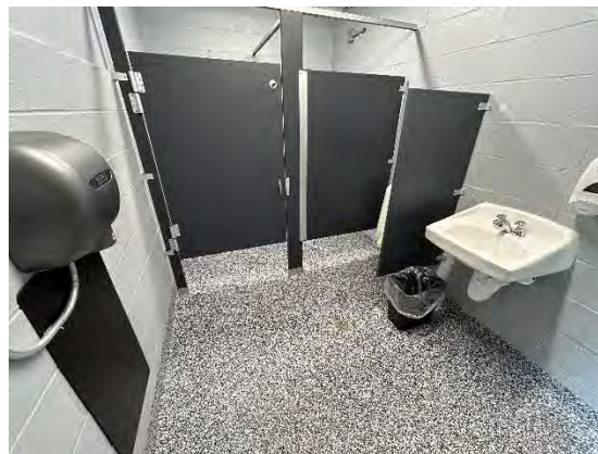
Northern Pavilion Left/East Toilet Room Interior
