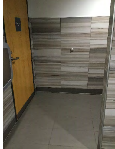
Terminal Men's Toilet Room Entrance Route
