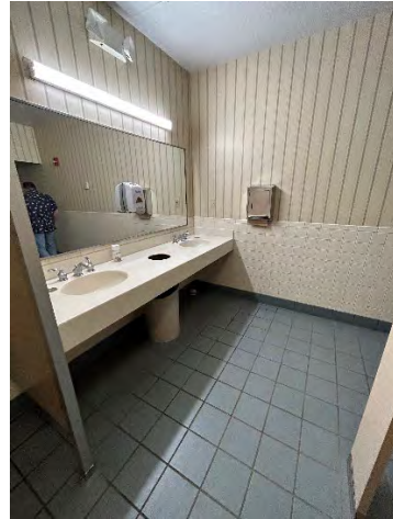
Men's Toilet Room Sinks
