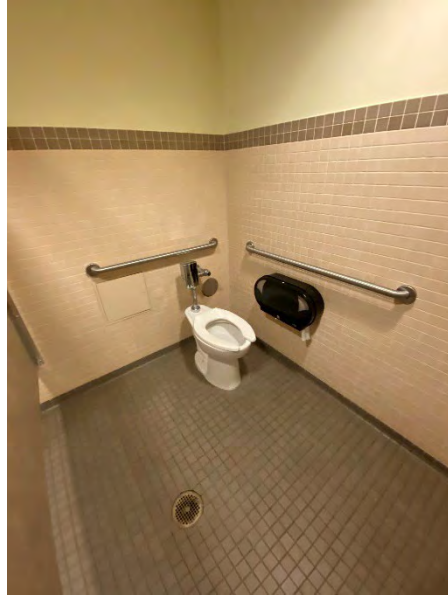
Men's Toilet Room Accessible Water Closet / Stall
