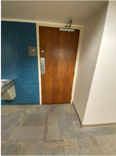
3 rd Floor Men's Toilet Room Entrance
