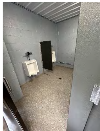
Pavilion #1 Men's Toilet Room Interior
