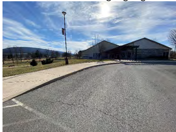
Exterior Entrance Route
