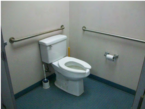
Toilet Room Accessible Water Closet / Stall
