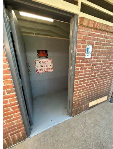
Pool Men's Toilet Room Entrance
