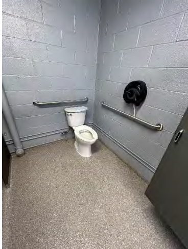
Pavilion #1 Men's Toilet Room Accessible Water Closet / Stall
