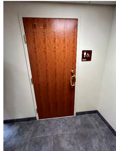
2 nd Floor Men's Toilet Room Entrance
