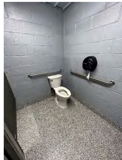
Men's Toilet Room Accessible Water Closet / Stall
