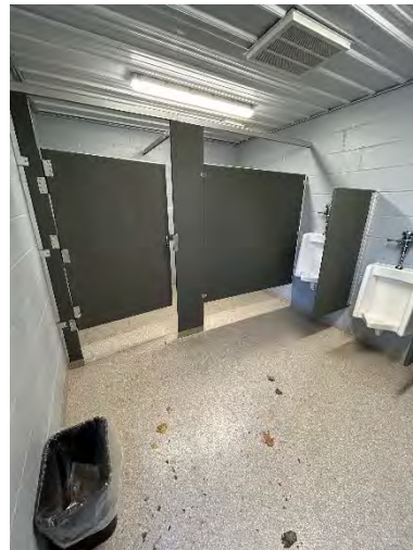
Men's Toilet Room Interior
