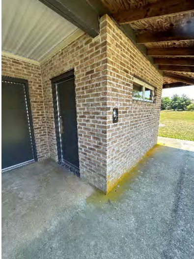
Upper Pavilion - Men's Toilet Room Entrance
