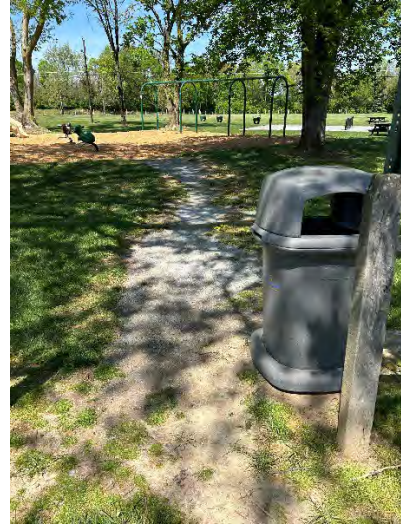
Exterior Accessible Route
