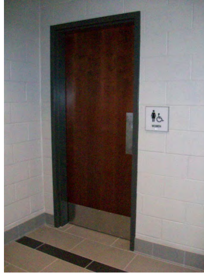
Women's Toilet Room Entrance
