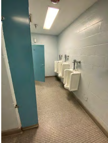
3 rd Floor Men's Toilet Room Interior
