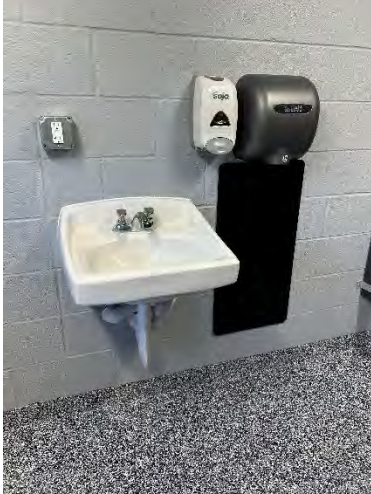
Pavilion #3 Men's Toilet Room Sink
