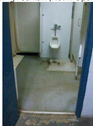
Toilet Room Interior
