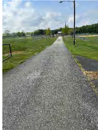
Exterior Entrance Route
