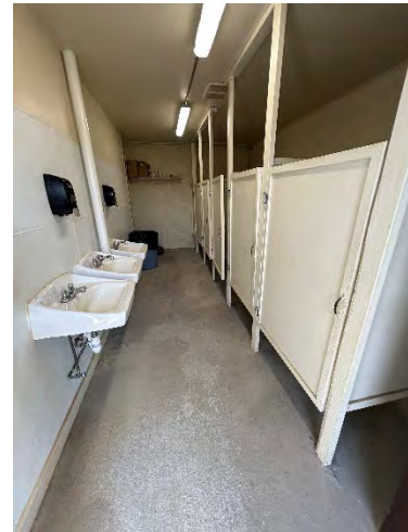
Women's Toilet Room Interior
