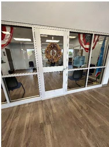
Entrance to Lobby
