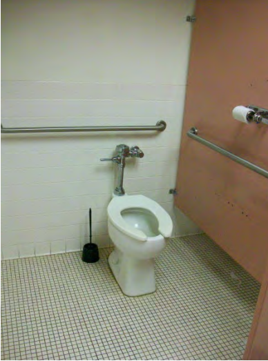
(Right) Women's Toilet Room Accessible Water Closet / Stall
