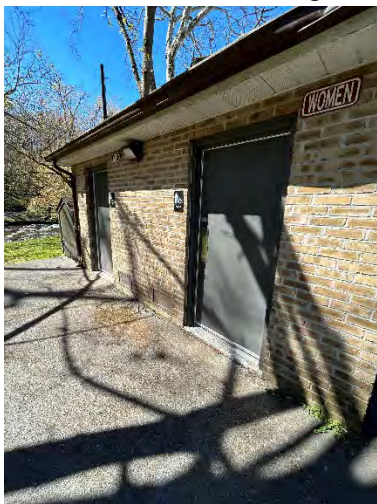
Toilet Room Entrances
