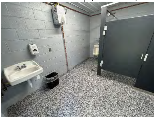
Arts Pavilion Men's Toilet Room Interior
