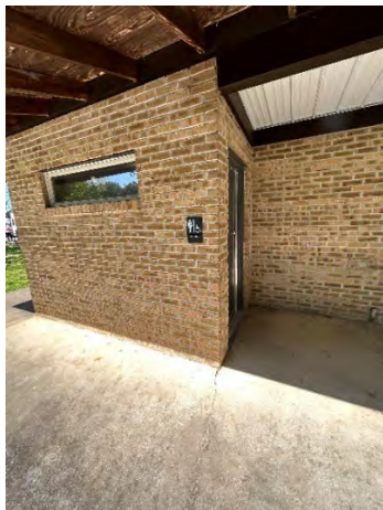
Pavilion #4 Women's Toilet Room Entrance
