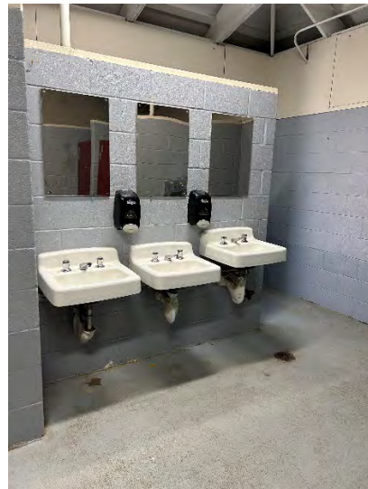
Pool Women's Toilet Room Sinks
