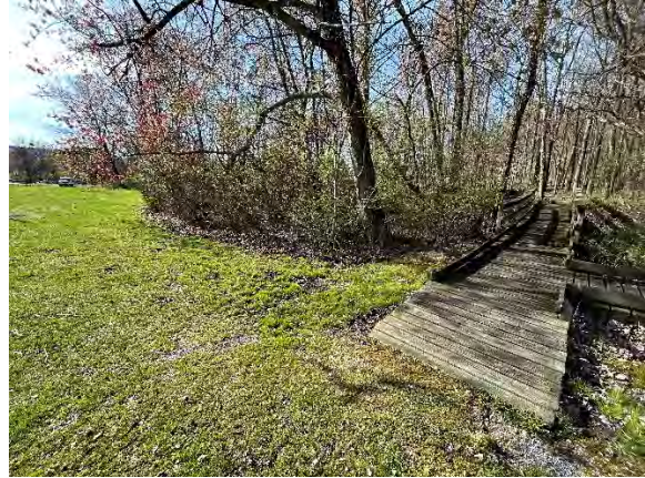
Exterior Access Route / Entrance to Elevated Walkway
