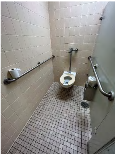
Women's Toilet Room Accessible Water Closet / Stall
