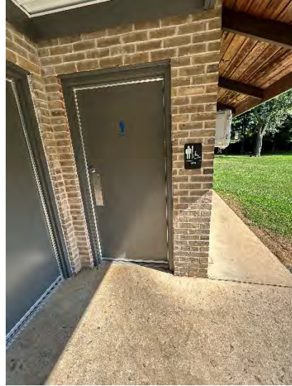
Pavilion #2 Men's Toilet Room Entrance
