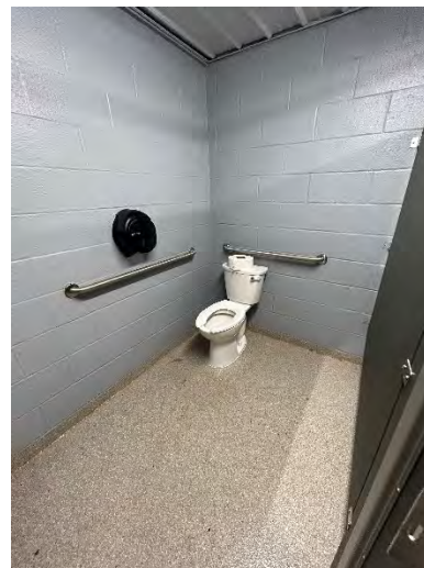
Men's Toilet Room Accessible Water Closet / Stall
