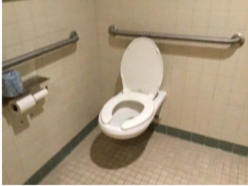
Men's Toilet Room Accessible Water Closet / Stall
