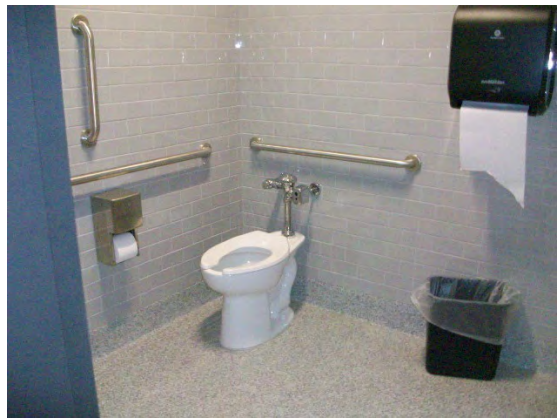
Staff Locker Room Single-Use Accessible Water Closet
