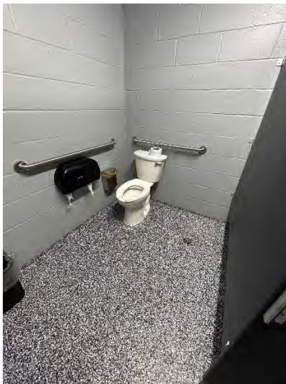
Pavilion #2 Women's Toilet Room Accessible Water Closet / Stall
