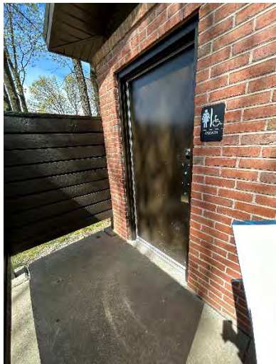
Women's Toilet Room Entrance
