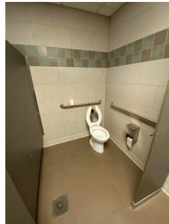
1 st Floor Men's Toilet Room Accessible Stall
