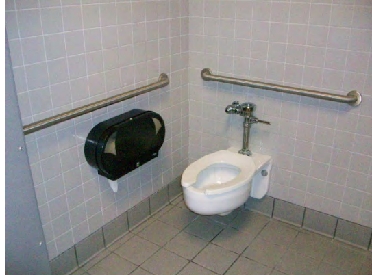
Men's Toilet Room Accessible Water Closet / Stall
