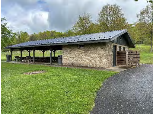
Pavilion / Toilet Rooms
