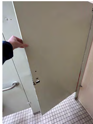
Women's Toilet Room Accessible Stall Door
