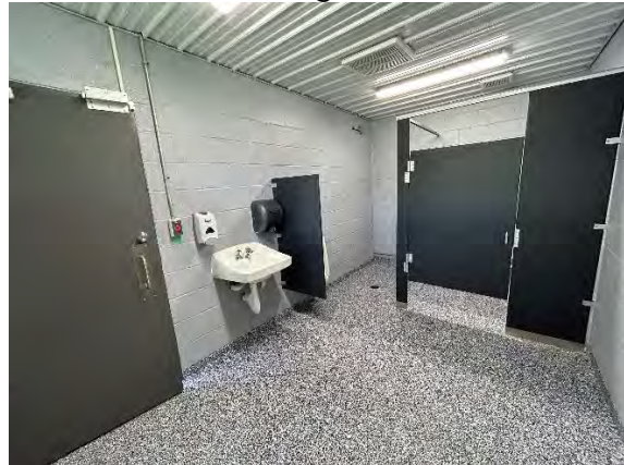
Lower Pavilion - Men's Toilet Room Interior
