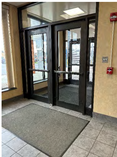
Main Entrance Interior
