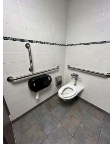
2 nd Floor Women's Toilet Room Accessible Water Closet / Stall
