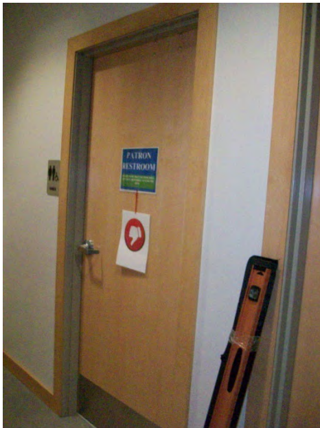
Single-Use Toilet Room Entrance
