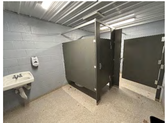
Women's Toilet Room Interior
