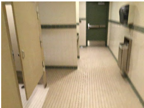
Men's Toilet Room Interior
