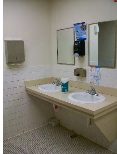
(Left) Men's Toilet Room Sinks
