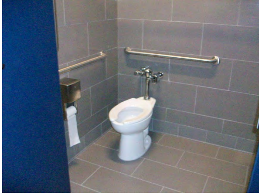
Men's Toilet Room Accessible Water Closet / Stall
