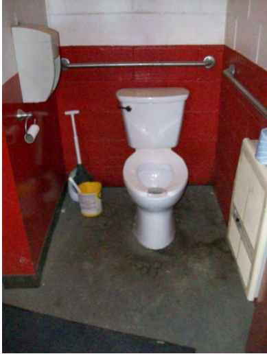
Toilet Room Accessible Water Closet
