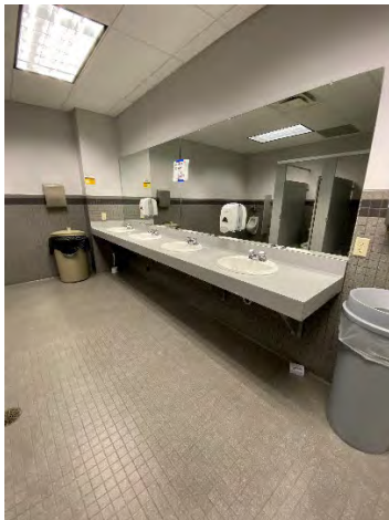
Men's Toilet Room Sinks
