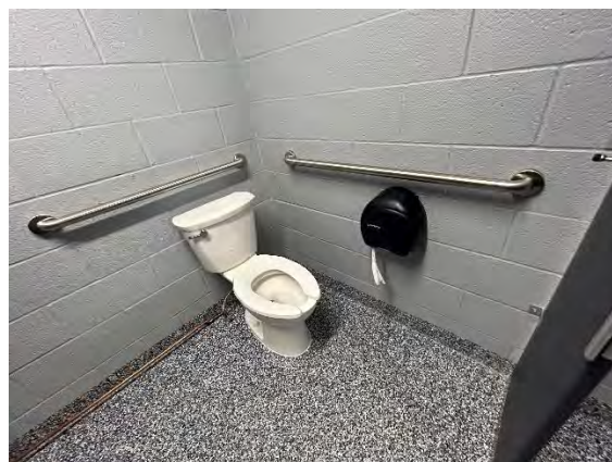
Men's Toilet Room Accessible Water Closet / Stall
