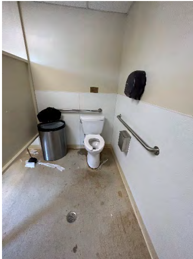
Women's Toilet Room Accessible Water Closet / Stall
