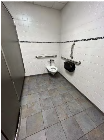
1st Floor Men's Toilet Room Accessible Water Closet / Stall
