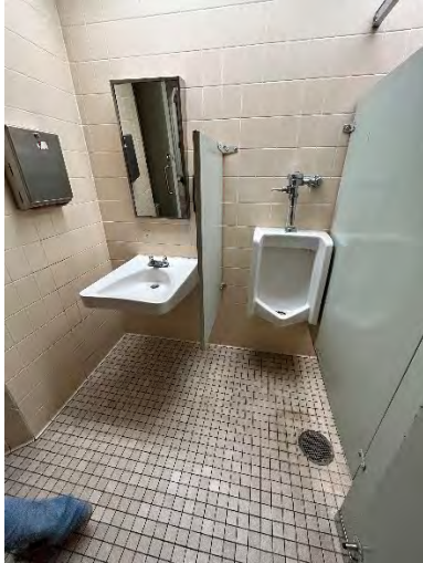
Men's Toilet Room Interior / Sink
