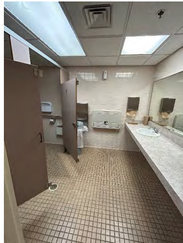
2 nd Floor Women's Toilet Room Interior
