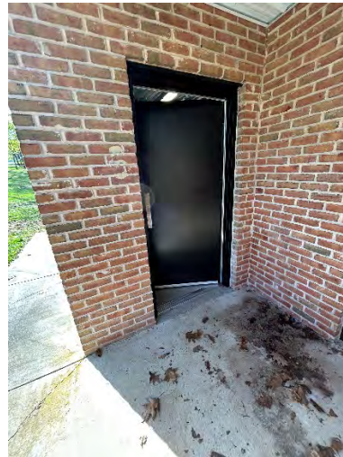
Pavilion #1 Women's Toilet Room Entrance
