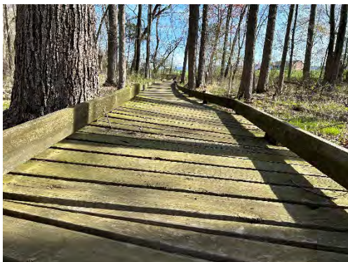
Elevated Walkway Surface
