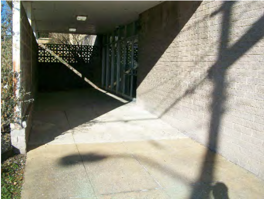
Exterior Entrance Route
