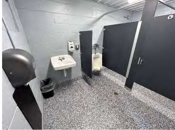
Southern Pavilion Right/South Toilet Room Interior
