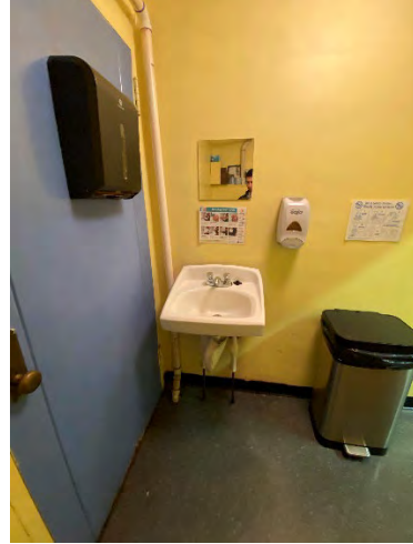
Single-Use Toilet Room Sink
