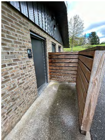
Women's Toilet Room Entrance
