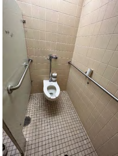
Men's Toilet Room Accessible Water Closet / Stall
