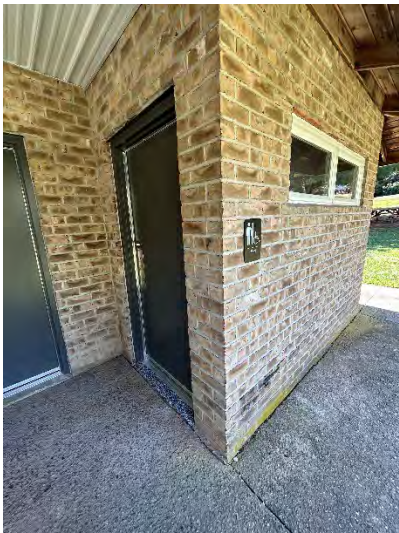
Lower Pavilion - Men's Toilet Room Entrance
