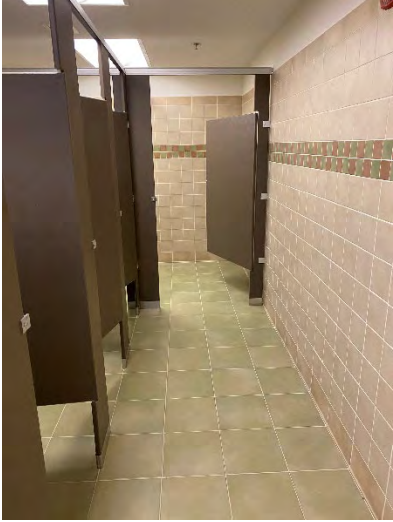
Women's Toilet Room Interior
