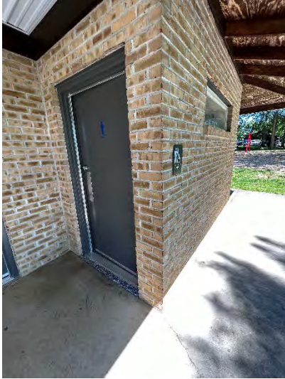
Pavilion #4 Men's Toilet Room Entrance
