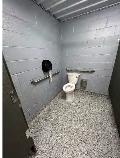
Women's Toilet Room Accessible Water Closet / Stall
