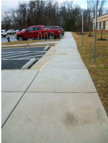
Exterior Entrance Route
