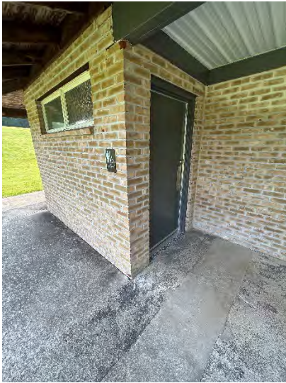
Women's Toilet Room Entrance
