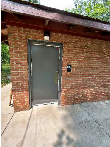
Southern Pavilion Right/South Toilet Room
