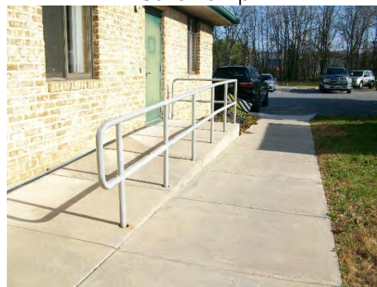
Ramp / Alternate Entrance
