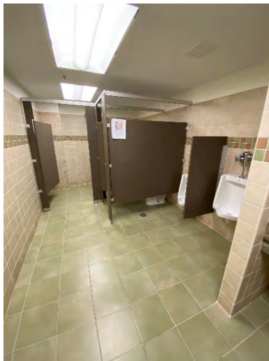
Men's Toilet Room Interior
