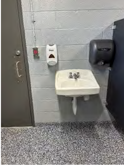
Lower Pavilion - Men's Toilet Room Sink
