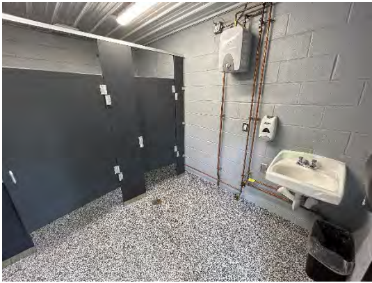
Arts Pavilion Women's Toilet Room Interior
