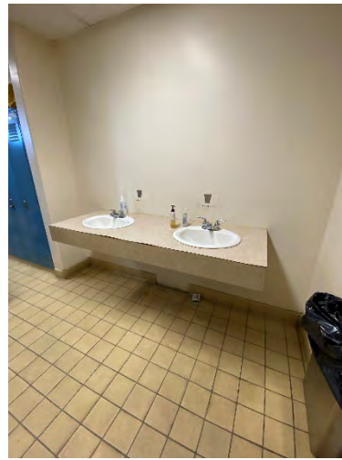
Men's Toilet / Locker Room Sinks
