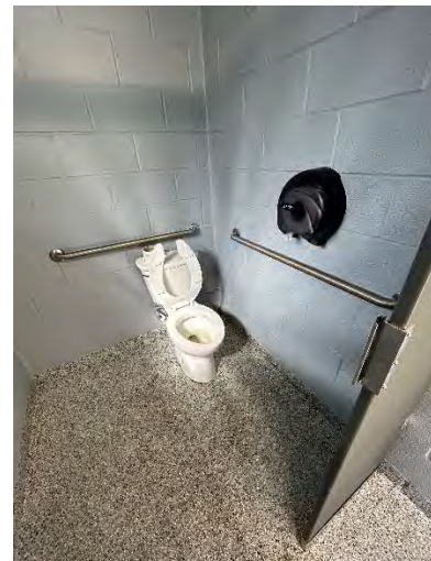
Men's Toilet Room Accessible Water Closet / Stall
