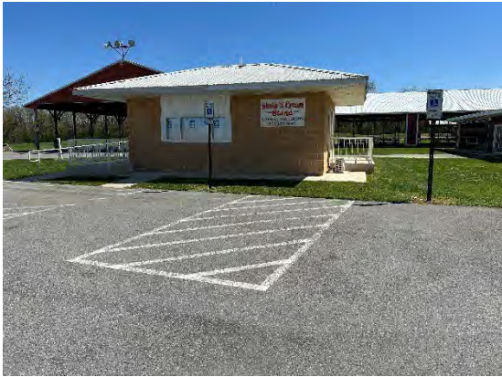
Accessible Parking / Concessions Building
