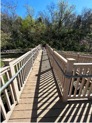
Top Portion of Ramp Entrance to Bridge
