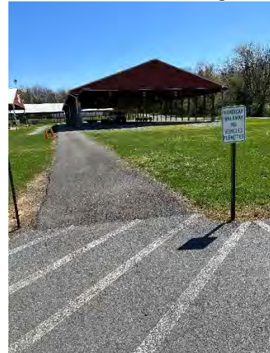
Exterior Accessible Route
