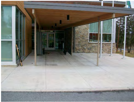
Exterior Entrance Route
