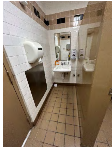
Rear Women's Toilet Room Sink
