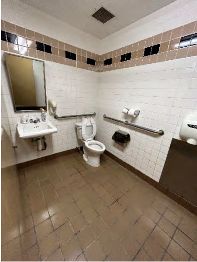
Rear Women's Toilet Room Accessible Stall
