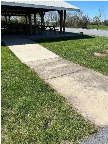
Exterior Accessible Route to Toilet Rooms
