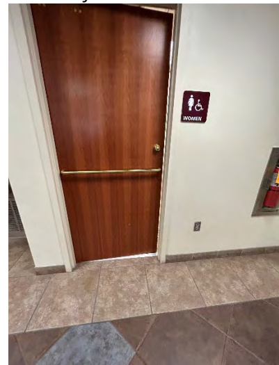
1 st Floor Women's Toilet Room Entrance
