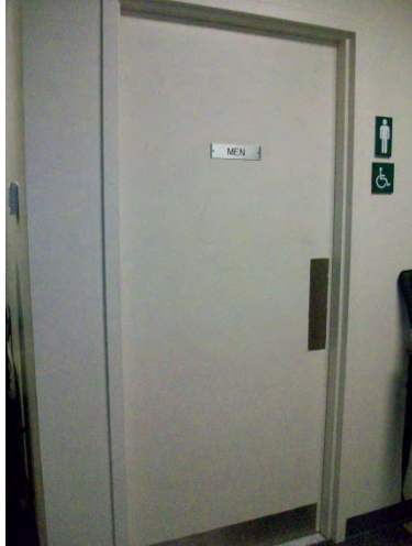
(Left) Men's Toilet Room Entrance
