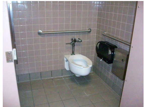
Women's Toilet Room Accessible Water Closet / Stall
