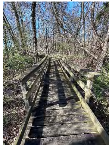
Elevated Walkway with Handrails
