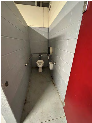
Pool Women's Toilet Room Accessible Water Closet / Stall
