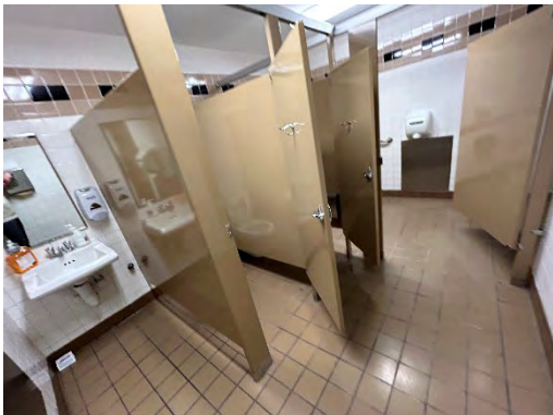
Rear Women's Toilet Room Interior
