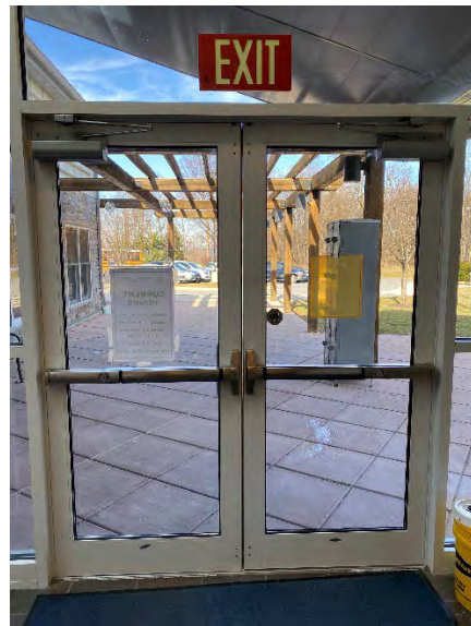
Main Entrance Interior
