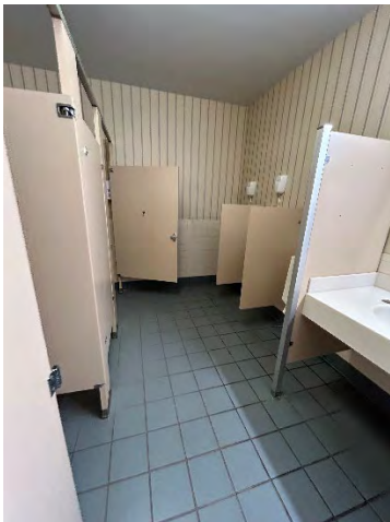
Men's Toilet Room
