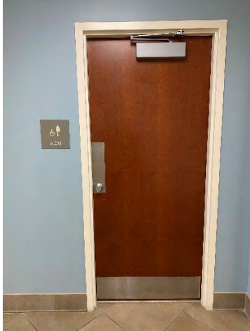
1 st Floor Men's Toilet Room Entrance
