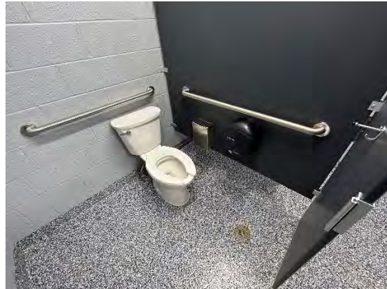
Women's Toilet Room Accessible Water Closet / Stall
