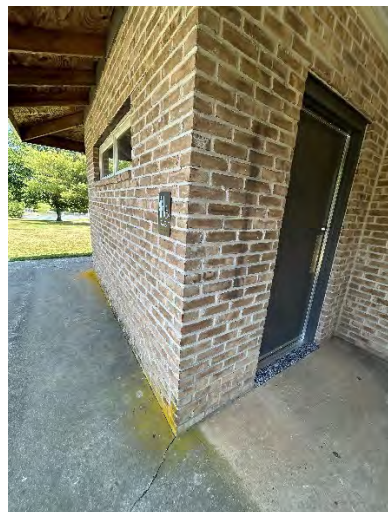
Upper Pavilion - Women's Toilet Room Entrance
