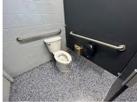
Pavilion #4 Women's Toilet Room Accessible Water Closet / Stall
