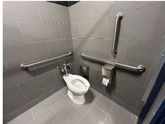
Women's Toilet Room Accessible Water Closet / Stall
