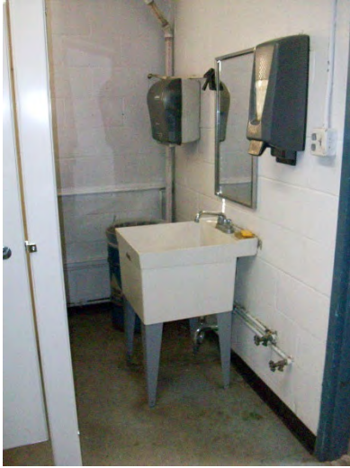
Toilet Room Sink
