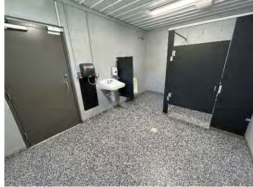
Upper Pavilion - Men's Toilet Room Interior
