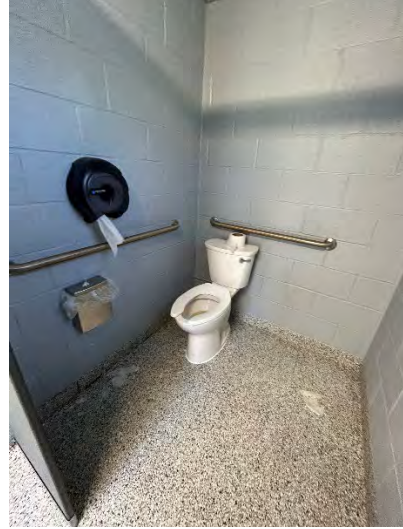
Women's Toilet Room Accessible Water Closet / Stall
