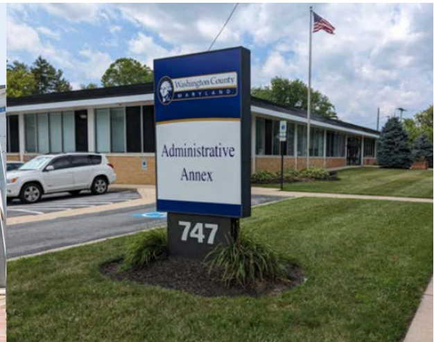
Administration Annex at 747 Northern Ave
