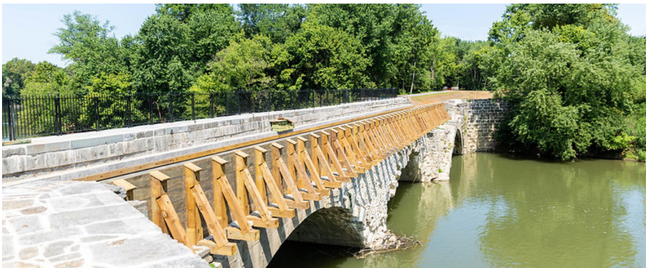
Conococheague Aqueduct, National Park Service
