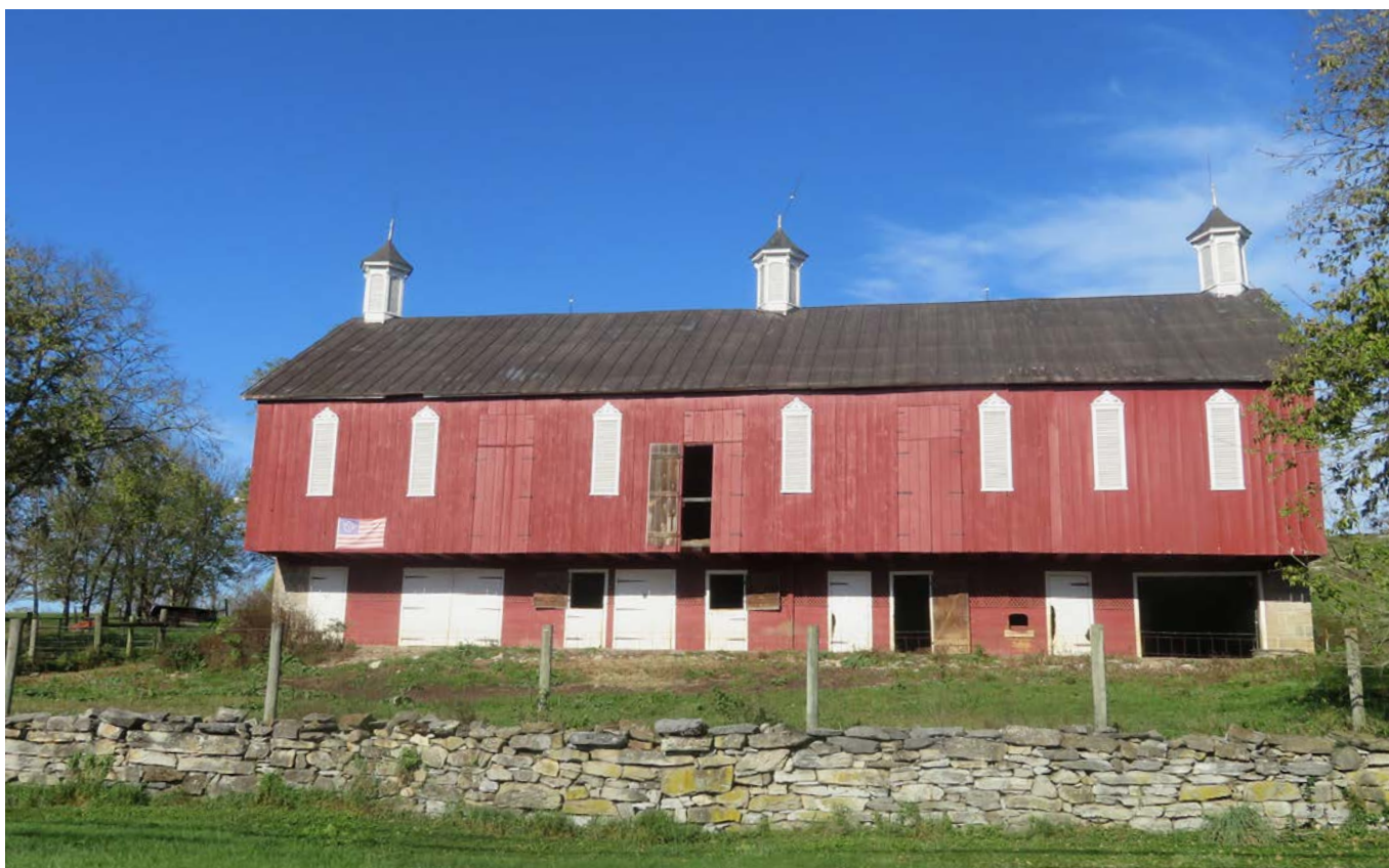
Farmstead, Wheeler Road, MIHP WA-II-286, Washington County Tax Credit and HP Overlay - Williamson
