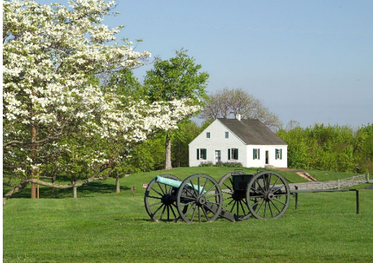
Dunker Church at Antietam National Battlefield
