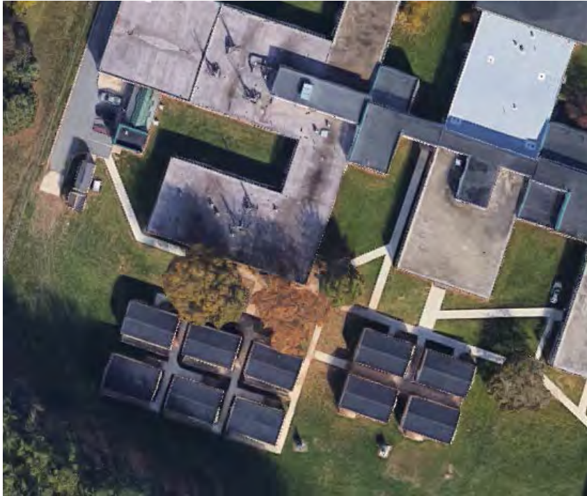
66 portables are located at 22 school sites
