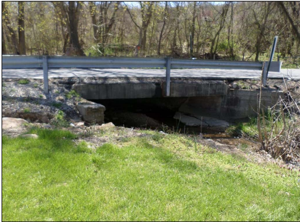
Trego Road Culvert 08/06
