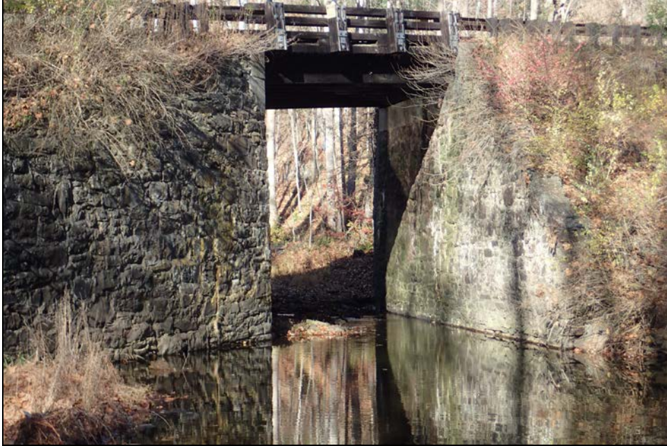
McFarland Road Bridge W002
