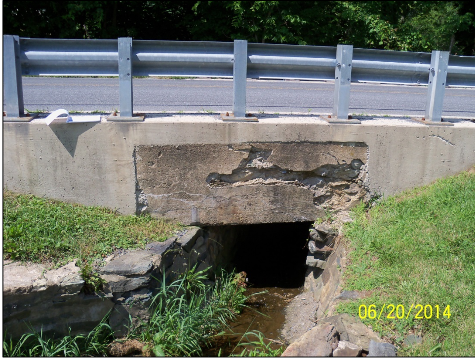
Trego Road 4000 Block Structure Repair
