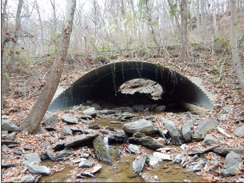
Burnside Bridge Road Bridge W5851
