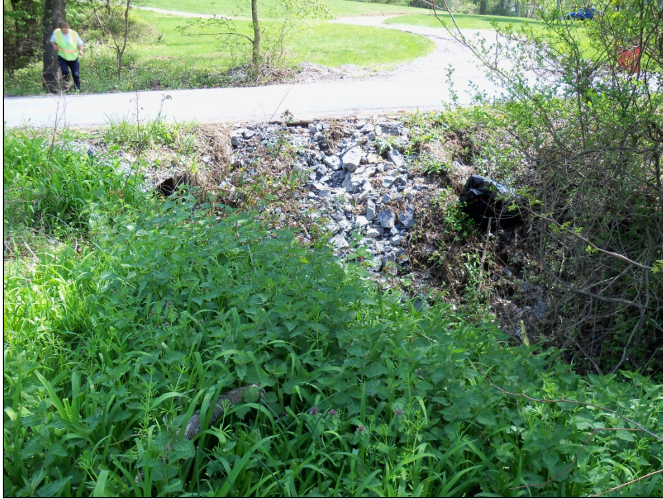
Trego Mountain Road North Culvert
