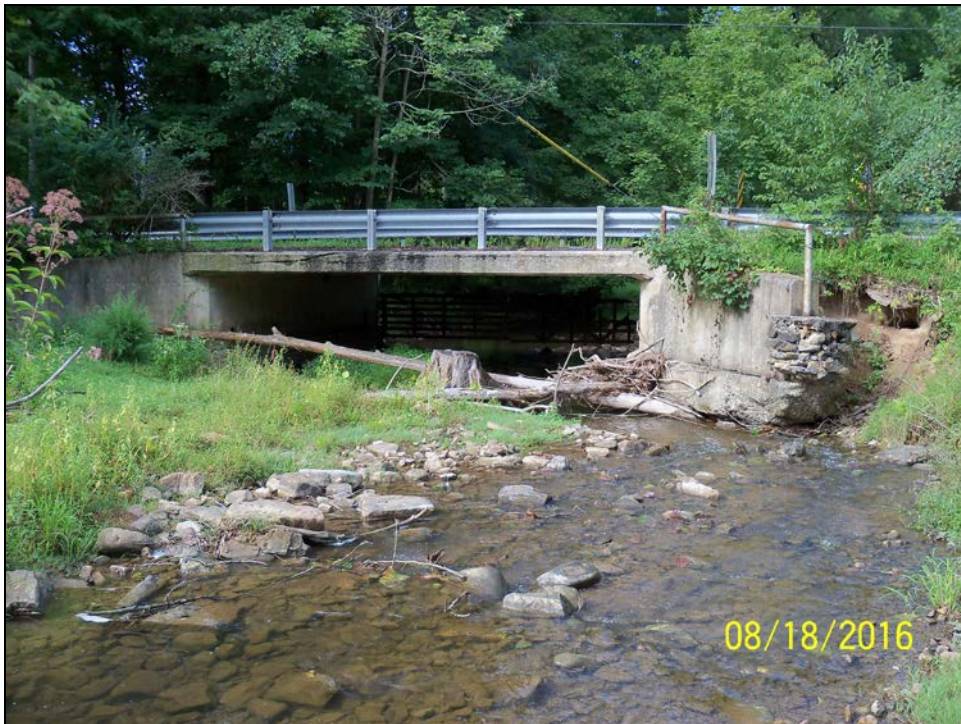
Licking Creek Road Bridge W0473
