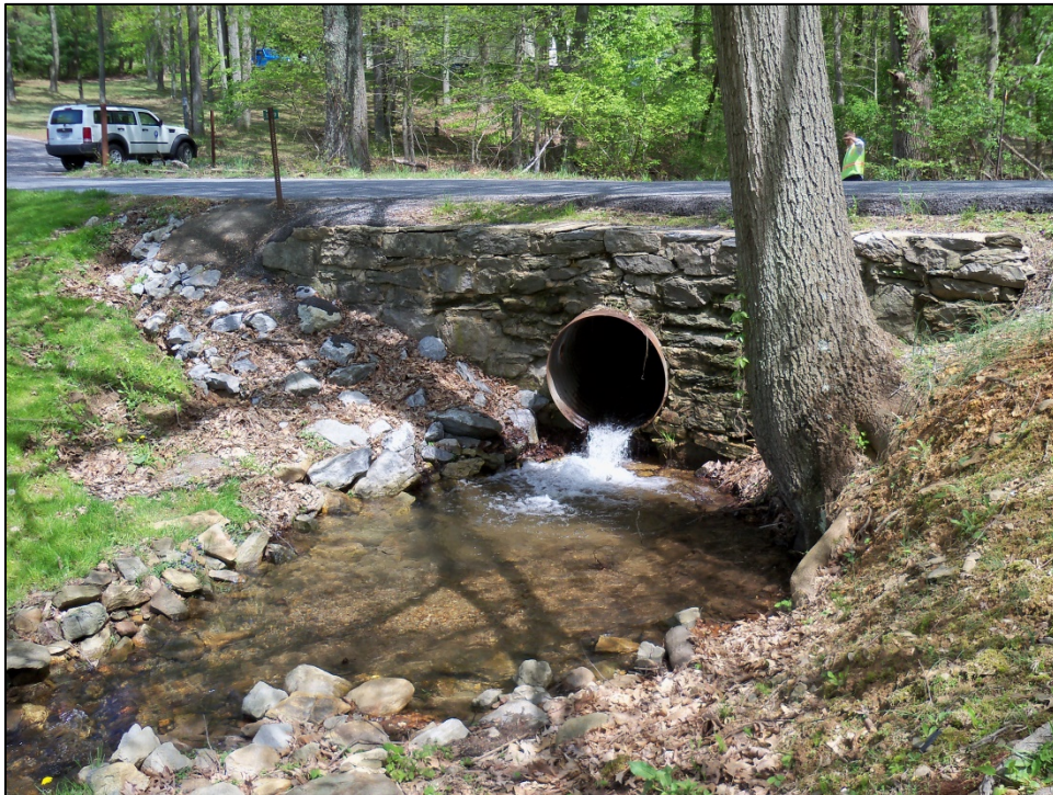
Trego Mountain Road South Culvert
